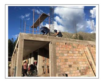
Hooray! The second floor of the Men's dormitory has begun as the rebars are now in place ready for the cement columns making possible the pouring of the roof.
