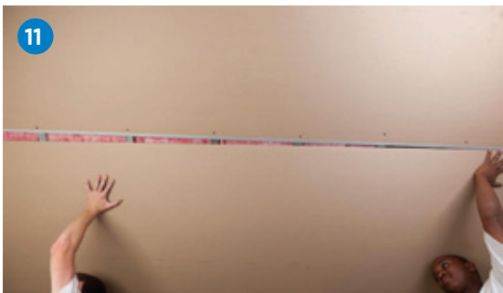
11 Install the next RhinoBoard 6.4mm. Repeat steps 9 and 10 until entire area is covered
