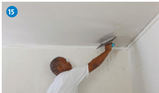
15 Using a 300mm steel trowel, scrap off the dead plaster (Fat).
