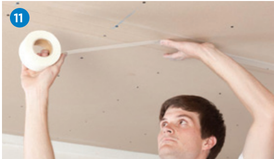
11 After boarding is complete, apply RhinoTape to all joints.
