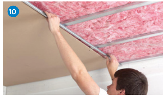
10 After installing the first board, measure and cut M-strip to size and install.
