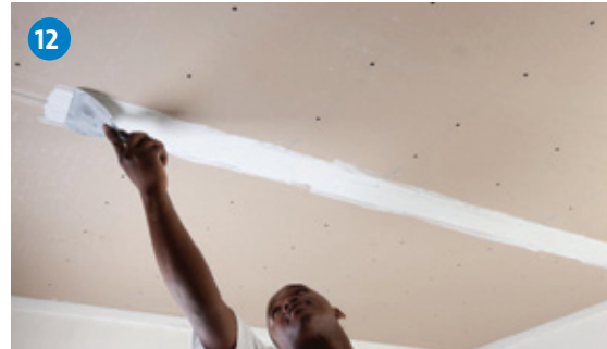
12 Apply Gyproc RhinoLite to all joints (pre-filling of joints) using a 150mm tapping knife.
