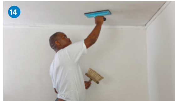
14 Leave the RhinoLite to set for a minimum of 40 minutes. Using a block brush lightly sprinkle water onto the RhinoLite surface. Use a sponge rubber float, and float the entire surface.
