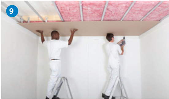
9 Measure and cut Gyproc RhinoBoard 6.4mm to size. Install the board and fasten using RhinoBoard Sharp Point Screws 25mm spaced at 150mm centres.
