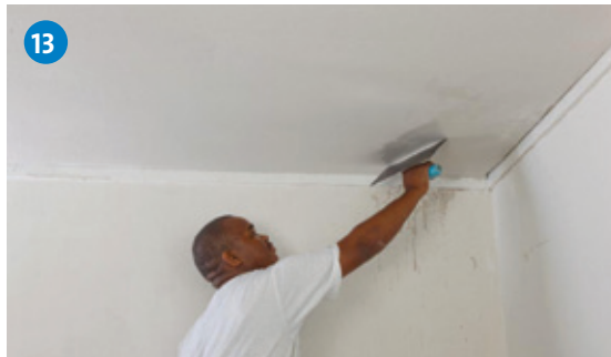
13 Apply RhinoLite to the entire surface using a 300mm steel trowel.
