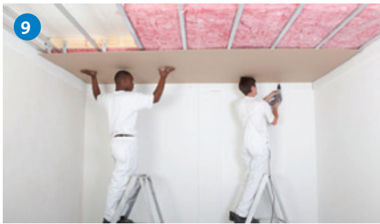
9 Measure and cut RhinoBoard 6.4mm to size. Install the board and fasten using Gyproc RhinoBoard Sharp Point Screws 25mm spaced at 150mm centres.
