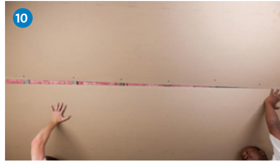
10 Install the next RhinoBoard 6.4mm. Repeat steps 9 until entire area is covered.
