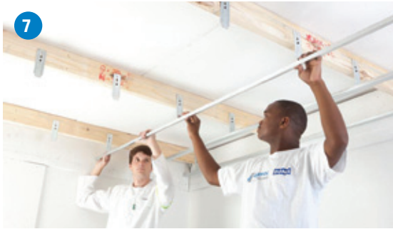
7 Measure and cut steel branding to size and clip onto suspension brackets.
