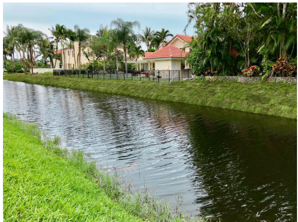
Erosion Control After
