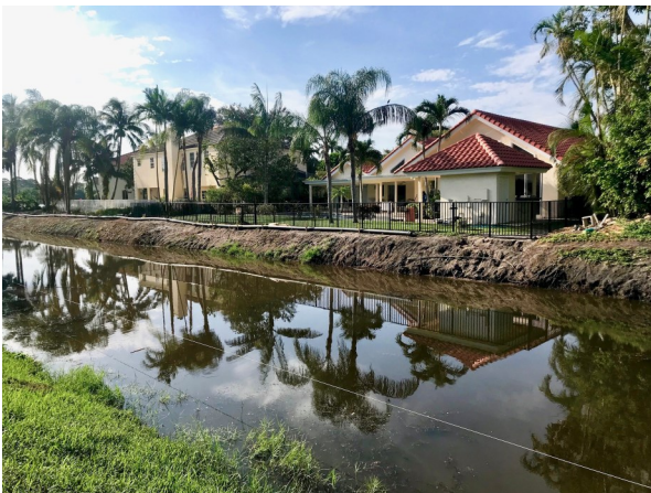
Erosion Control Before
