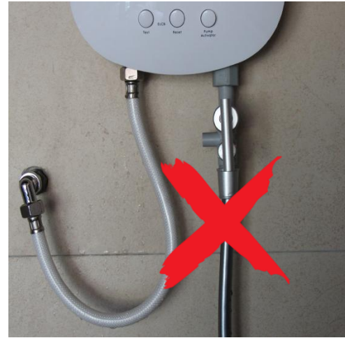
Stop valve installed at outlet (Close outlet)
