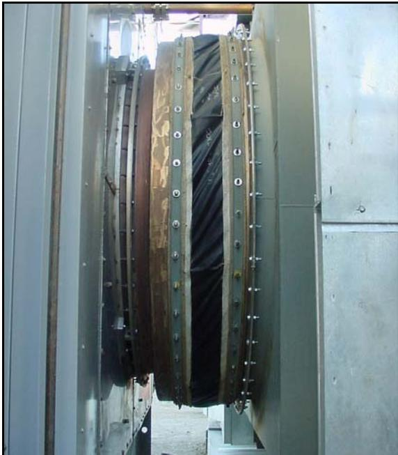
Ø89 inch diameter Gas Turbine Exhaust Expansion Joint with Hot to Cold Frame. 25 in wc at 980°F.
