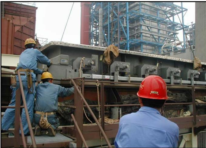
FGD Tandem Bypass Damper being installed in China
