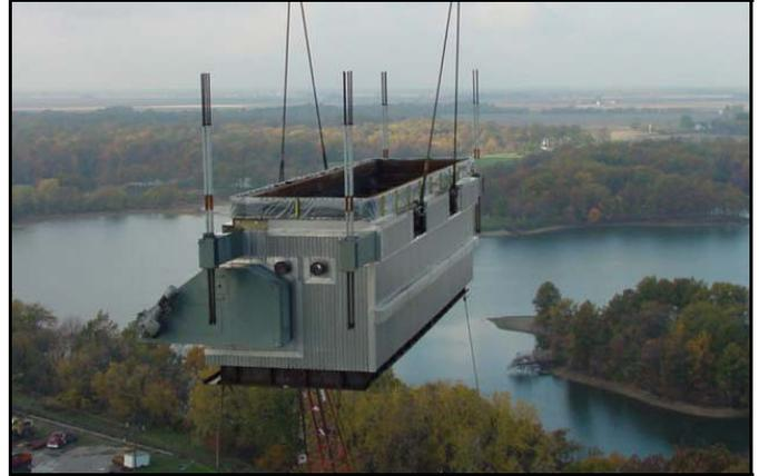
SCR 4-port diverter module being lifted into place in the United States
