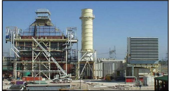
GT Exhaust System being installed in Argentina
