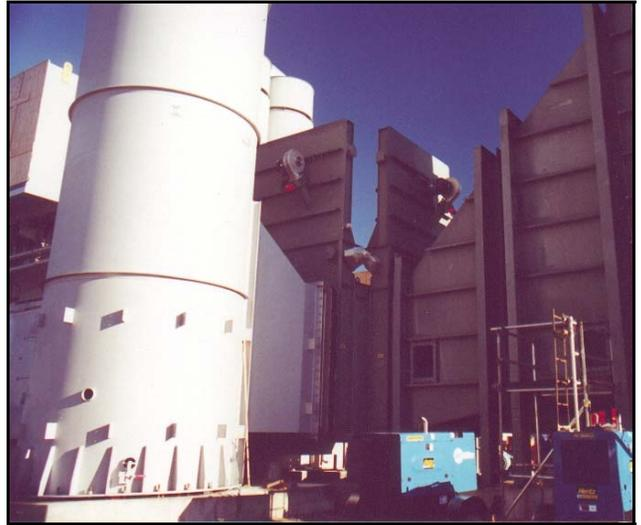
GT Guillotine Bypass System for GE LM6000 in Canada
