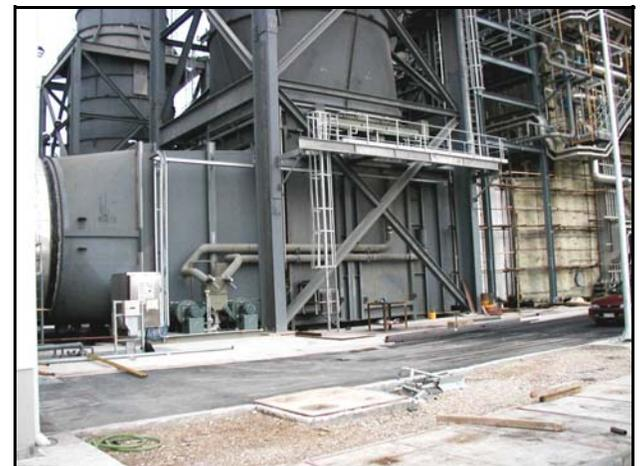
GT Diverter Bypass System for Alstom GT13E2 in Greece
