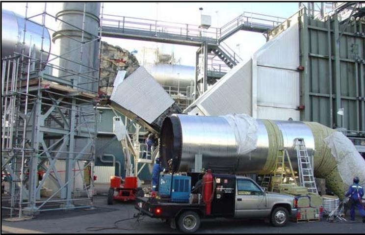
Bachmann Field Service Personnel assisting with the installation of a gas turbine expansion joint.
