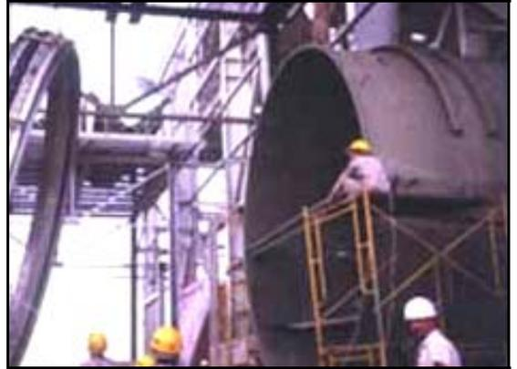
Ø120 inch diameter Gas Turbine Expansion Joint during installation. 25 in wc at 1070°F.
